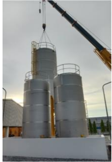
Stainless steel 304 DOA Storage Tank, Size 34 m 3
